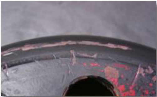
Scratch in guide wheel shell sealing area
