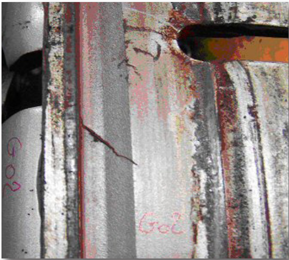
Crack in the rim flange
