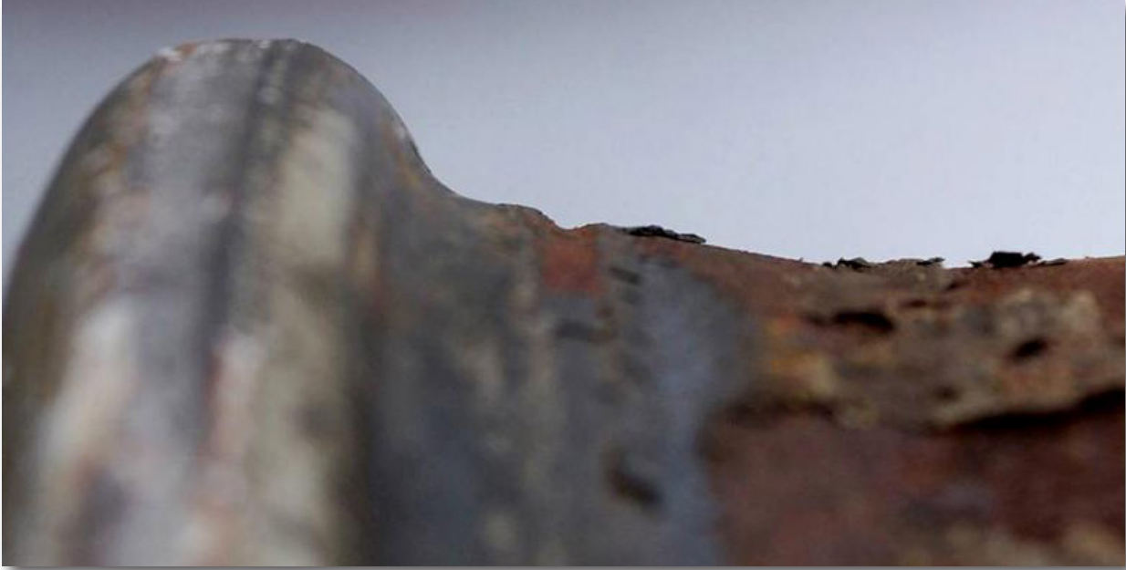
Wear on the seat due to corrosion and overloading
