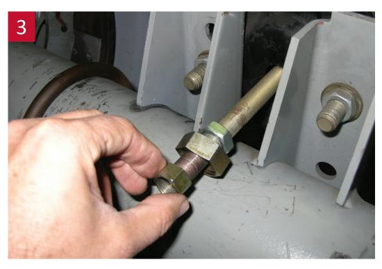
When installing a Gunite slack adjuster with a collar lock clevis, place the 1-1/4" collar nut on the push rod against the 15/16" jam nut. Next thread the <sup>3</sup>/<sub>4</sub>" hex nut onto the push rod.
