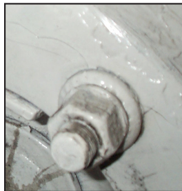
Visible signs that paint exceeds the maximum allowable thickness of 3.5 mils. Multiple coats, uneven surfaces, and illegible stampings indicate too much paint.
