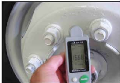
Paint thickness gauge reads 16.68 mils, above the maximum allowable thickness of 3.5 mils.
